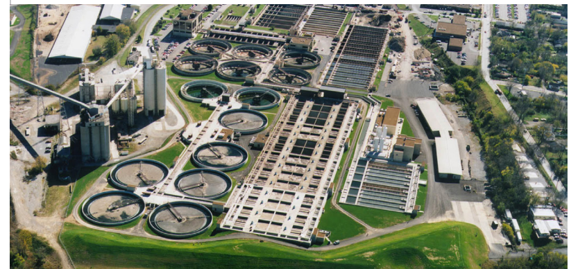
SEWERAGE TREATMENT FACILITY
